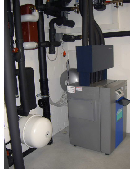
Figure 8. Private home equipped with heat pump for heating and active cooling (brine/water heat pump with transformer box to switch automatically from heating to cooling mode and inverse. Cooling power is 14.4 kW (at +8/+35 °C).
